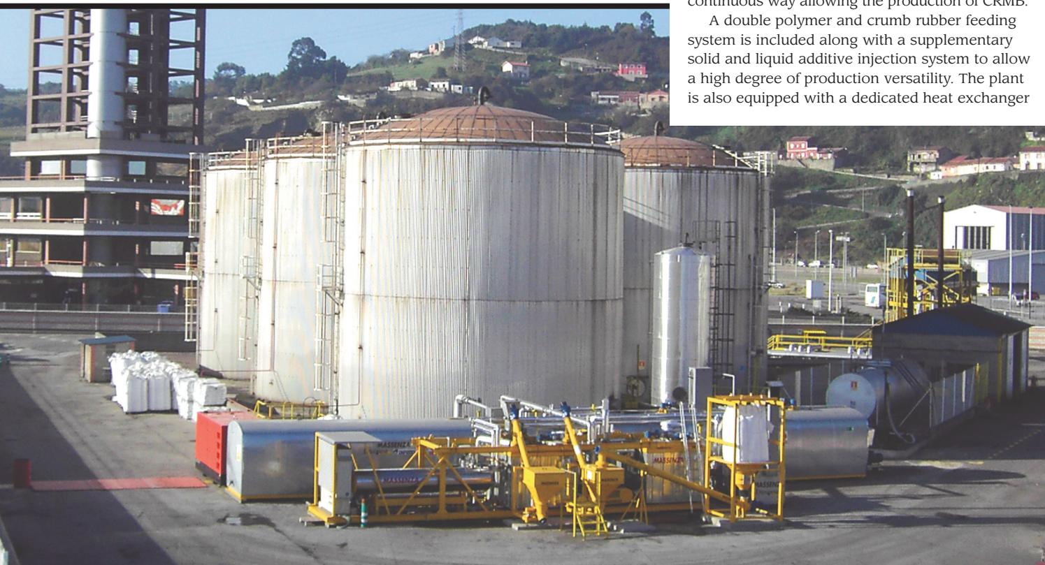
for instantaneous heating up of bitumen during loading; bypass valve for homogeniser and pumps with variable frequency drive to manage PMB or CRMB production; complete automatic production cycle managed by PLC and touch screen and a full set of ancillary equipment including storage tank for neat bitumen, digestion tank for modified bitumen and thermal oil heater.
